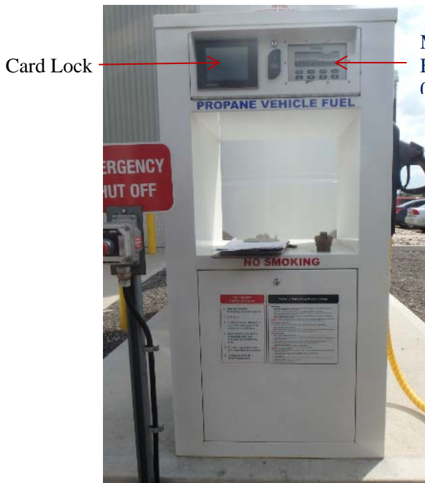
Figure 6: Propane dispenser (front view) / Distributrice de propane (vue de face)
