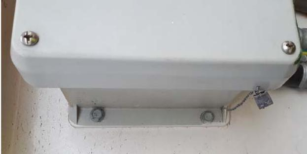
**Sealing of junction box, with two diagonally opposed cover seals /
