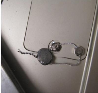
**Typical wire and seal method for
