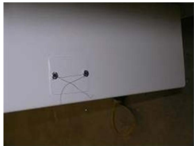
Typical sealing of the cover plate/ Scellage typique de la plaque d'acier
