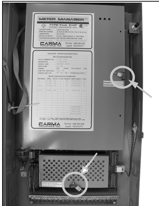
Rev. 14 Sealing of Meter Manager type T/mA Rév 14 Scellage de Meter Manager type T/mA
