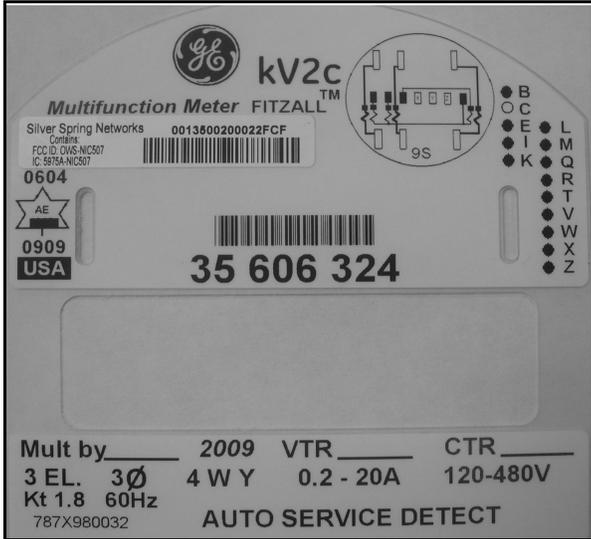
**kv2c markings with new SSN module /
