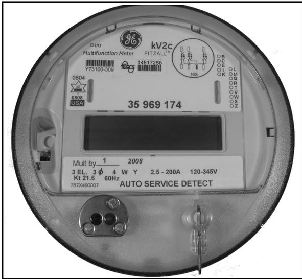
**Nameplate for UMT-C-KV with EMTR-3-KV /
