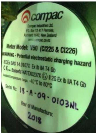
Figure 3 Sample nameplate for meter |
