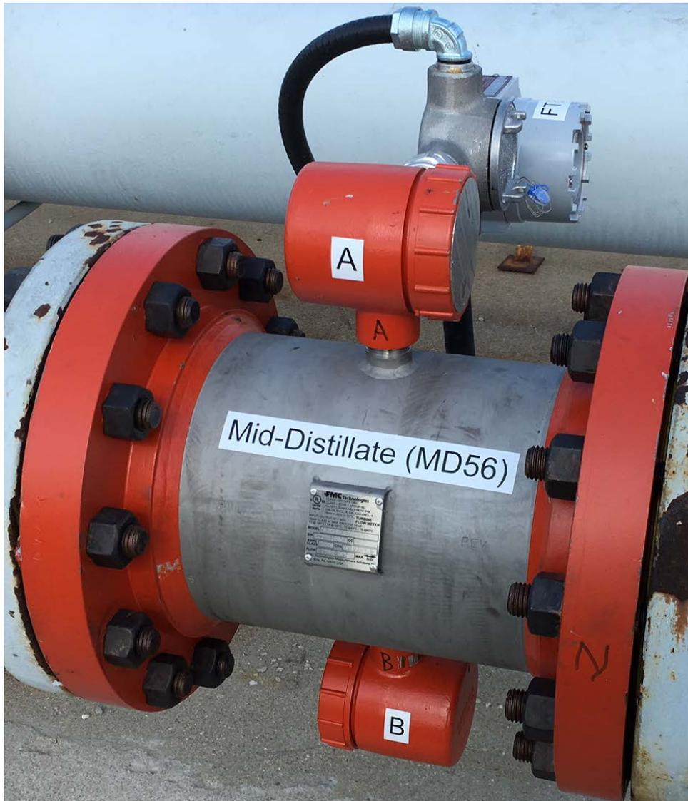
Figure 1: The K2D 8 Inch Sentry Turbine meter with two pickup coils |
