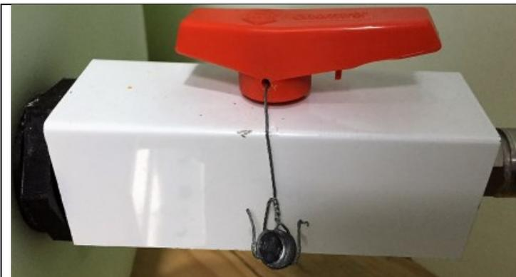
Figure 10 Sealing the Low-level inspection valve |
