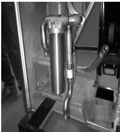
Check valve/Clapet de retenue
