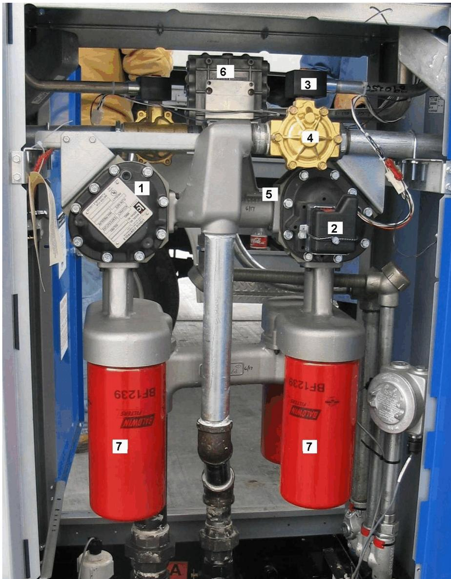
**Fig. 6: Hydraulic structure of UHC dispensers /
