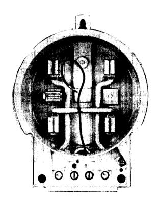
Another jumper joins the two inner terminals and is provided with a short potential lead terminated with a clip for attaching it to the RH test link.
