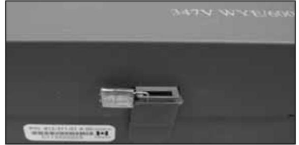
**Voltage Transformer Utility Sealing Location /
