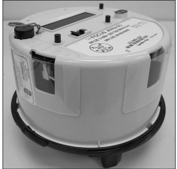
**Polycarbonate shields placed over the meter housing
